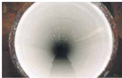
FER-PAL Infrastructure uses innovative technology called Aqua-Pipe, which allows pipes to be refurbished in place without having to be dug up. SUPPLIED
